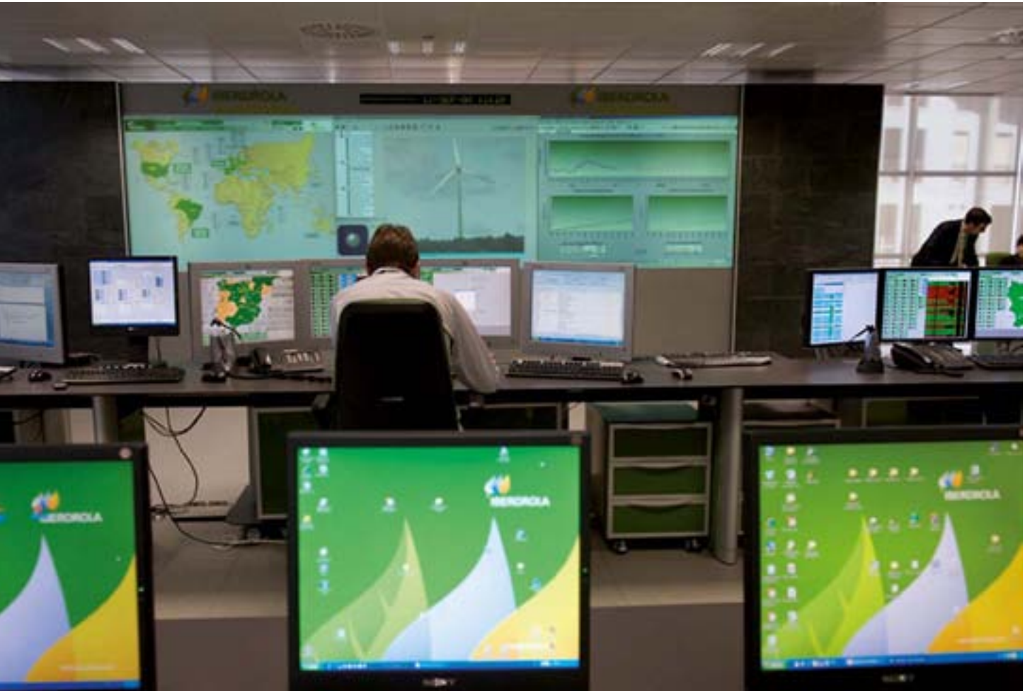
Iberdrola control center, Spain © Wind Power Works
