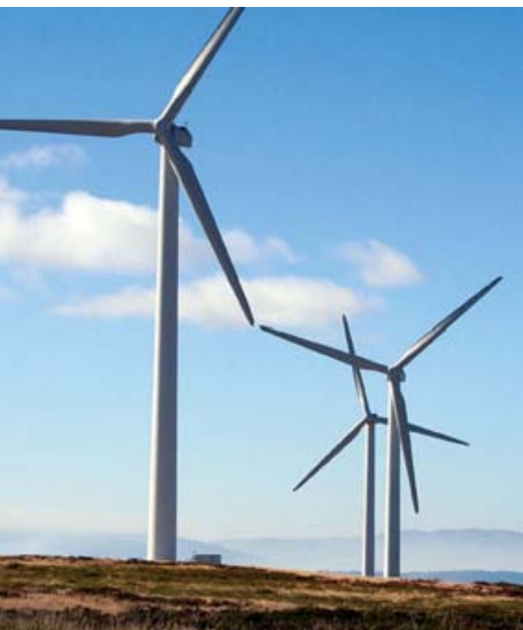
Cabeço Alto wind farm © Nordex Energy
